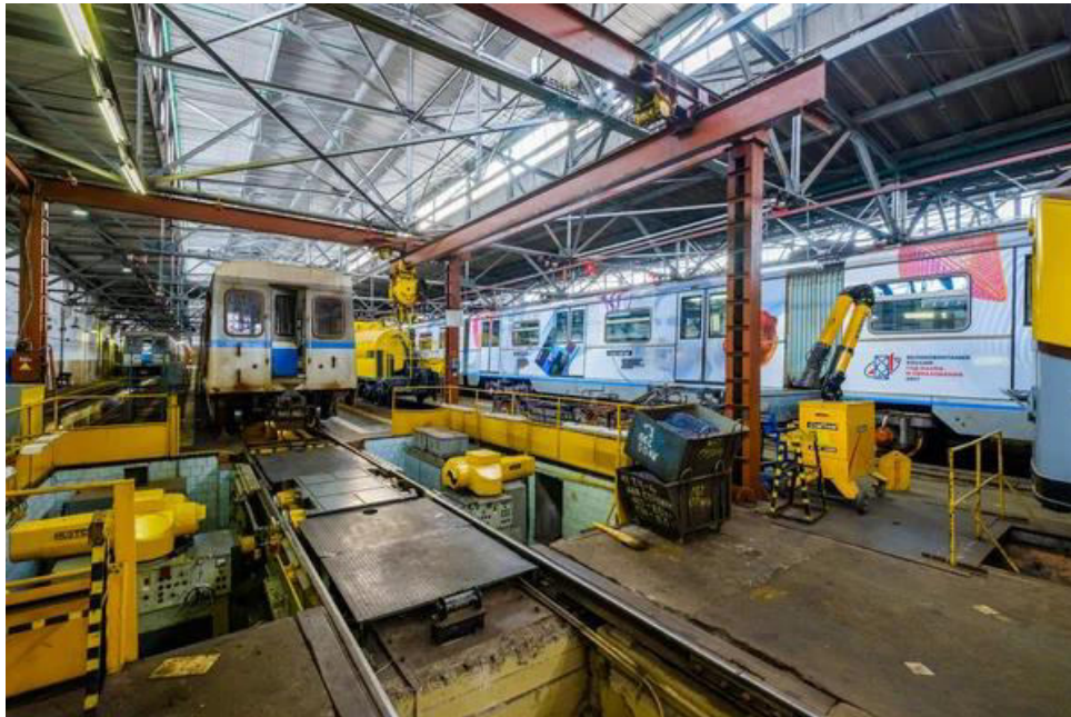
Figure 2: Locomotive and Wagon Workshop, Rostov, Russia Federation
