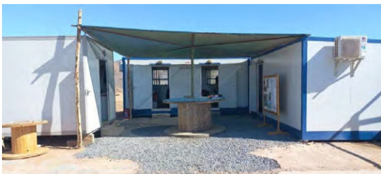
Photo 9 – View of site offices kept neat and tidy. Entire site is well maintained and kept in perfect condition.
