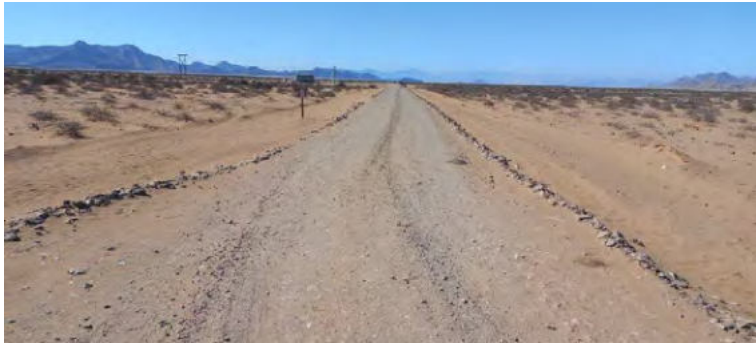
Photo 21 – View of access road in between the Contractor's Offices- and the construction site. Road is well maintained and earmarked.
