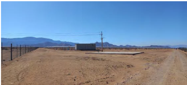
Photo 23 – View of E-house and OHTL on the construction site.
