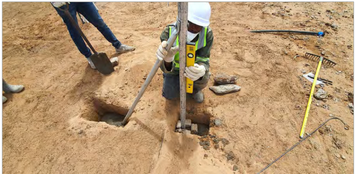
Figure 4 - Installation of the fence.
