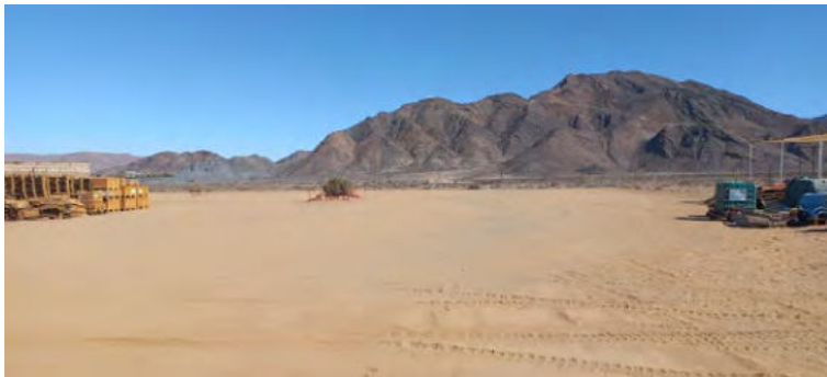
Photo 11 – View of Contractor's site. Neat, organised and well maintained.
