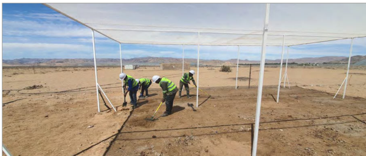
Figure 2 - Nursery area cleaning process.
