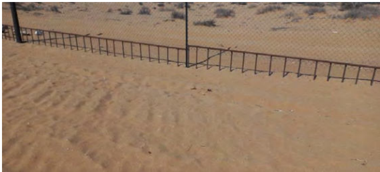
Photo 26 – View of open space at bottom of boundary fence to provide for natural storm water flow and small mammal, reptile, etc. movement.
