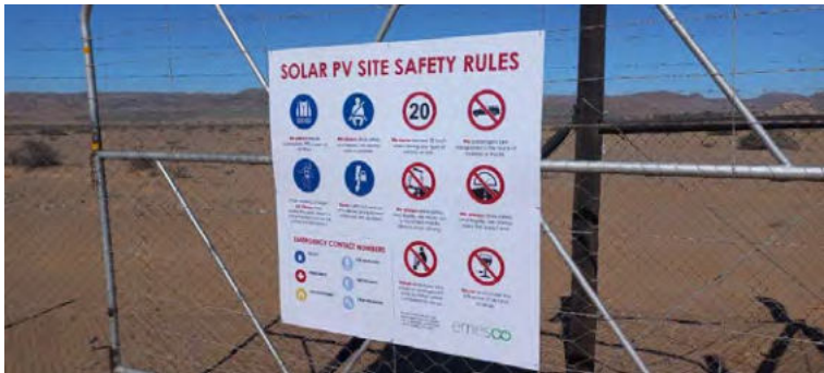
Photo 22 – View of information board at entrance to the construction site. All requirements in accordance with health and safety is covered by the sign.
