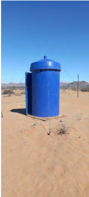
Photo 28 – View of on-site toilet, secured to the ground. On-site toilets are clean and well maintained.
