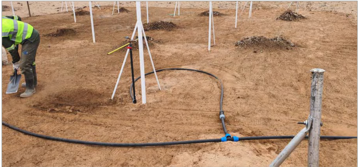
Figure 3 - Installation of water line.
