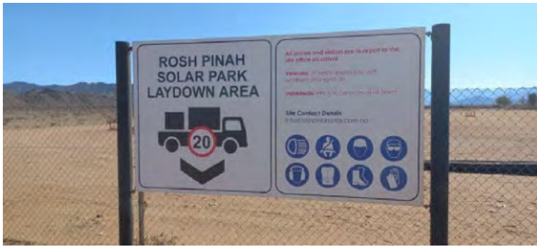
Photo 4 – View of sign at the entrance to the Site Office indicating the dedicated laydown area with required safety requirements to access the site. Sign is visible and well maintained.
