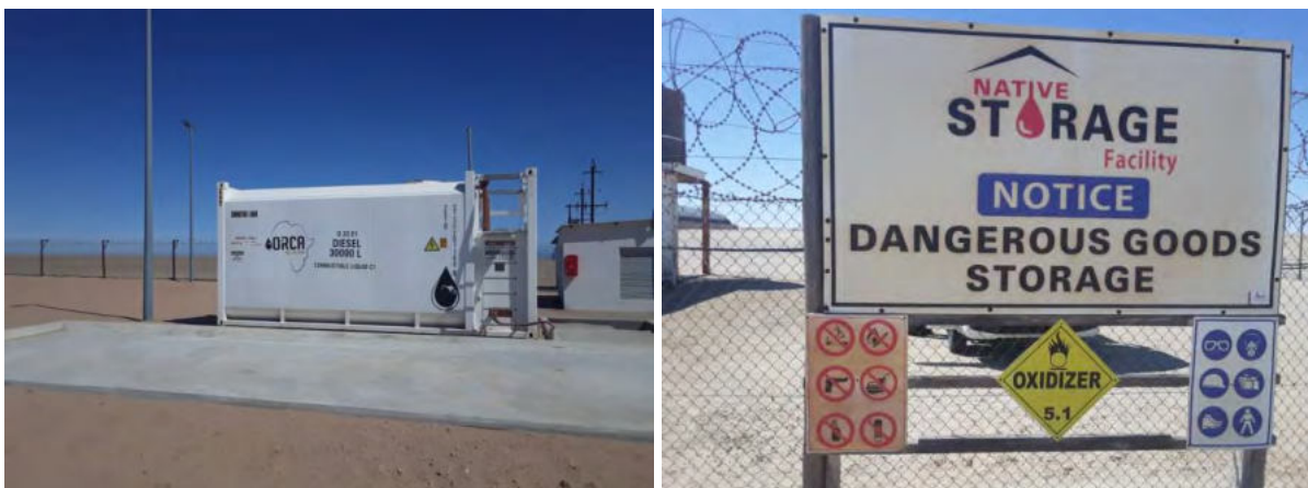
Figure 3: Self-bunded Diesel Fuel Tank and Signage
