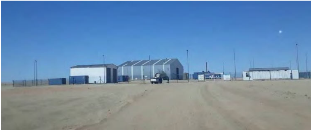
Figure 4: Ammonium Nitrate Emulsion Production Facility
