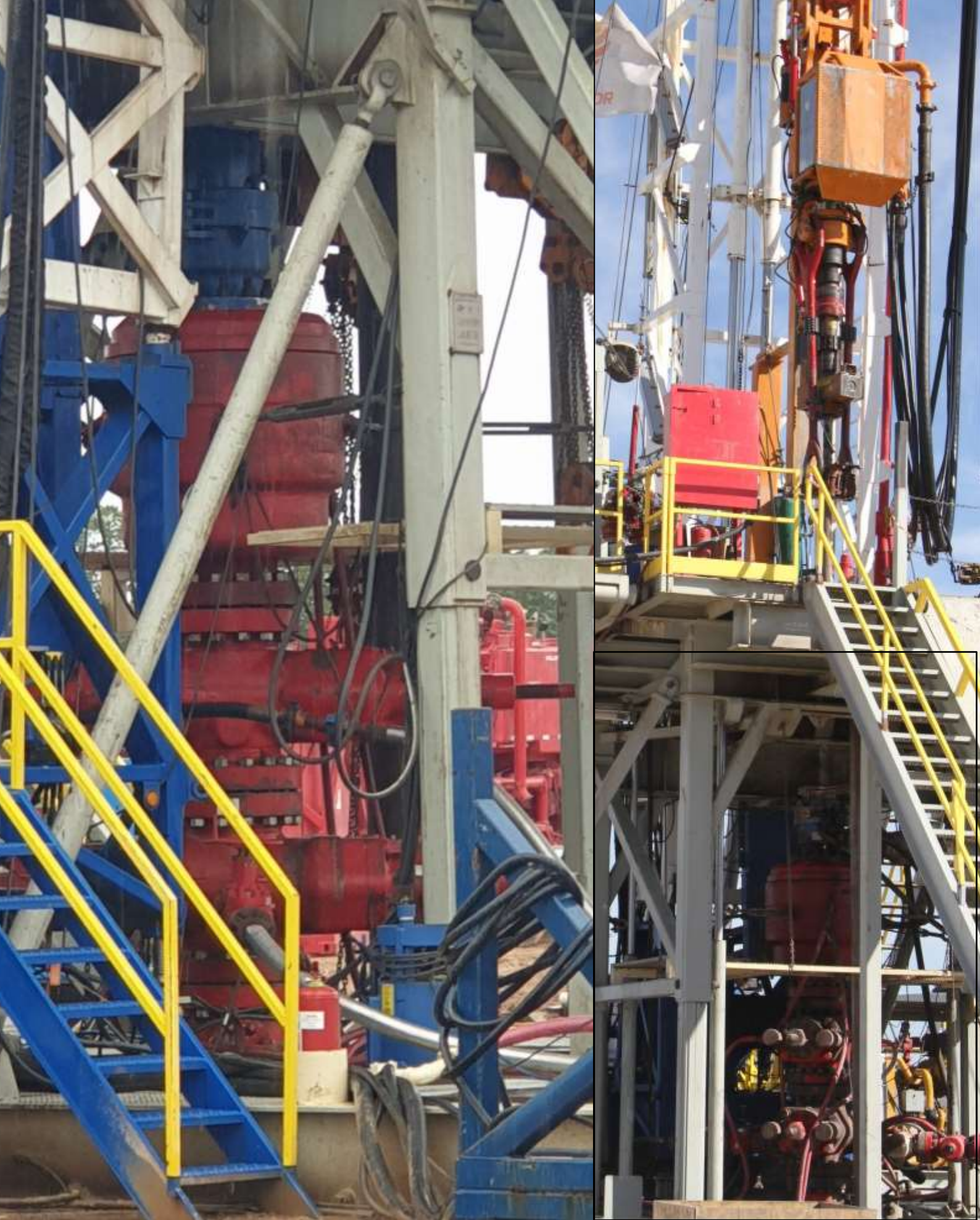
Plate 4.1: BOP stack used in the drilling of the proposed exploration and appraisal wells Nos. D1-D6 and G1-G6 within the AOI in PEL No. 73.
