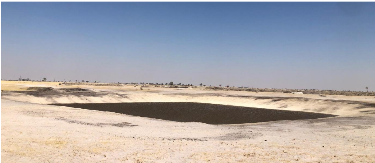
Figure 2-2: Oshihe earth dam site
