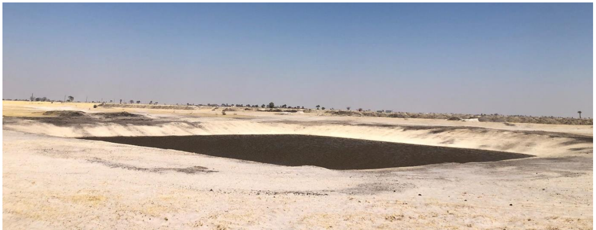
Figure 2-2: Oshihe earth dam site
