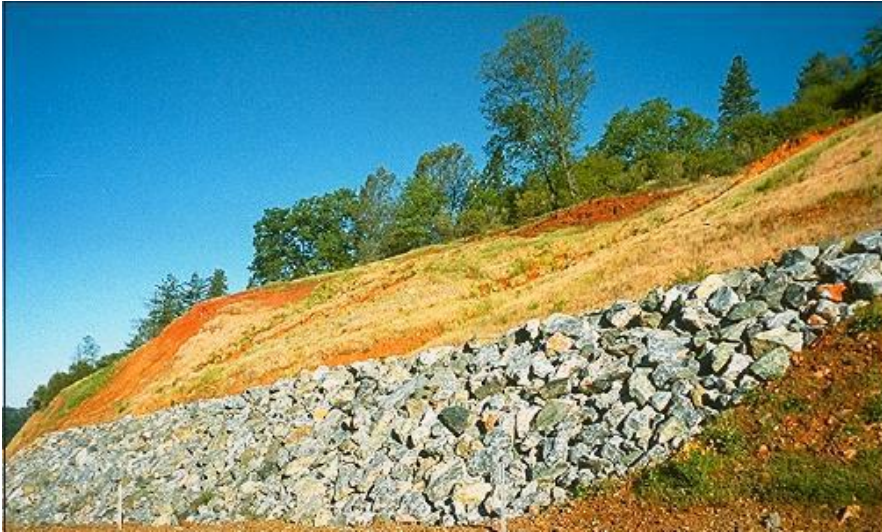
Figure 2-4: Rock buttress illustration
