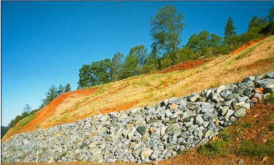
Figure 2-3: Rock buttress illustration
