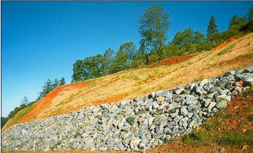
Figure 2-2: Rock buttress illustration
