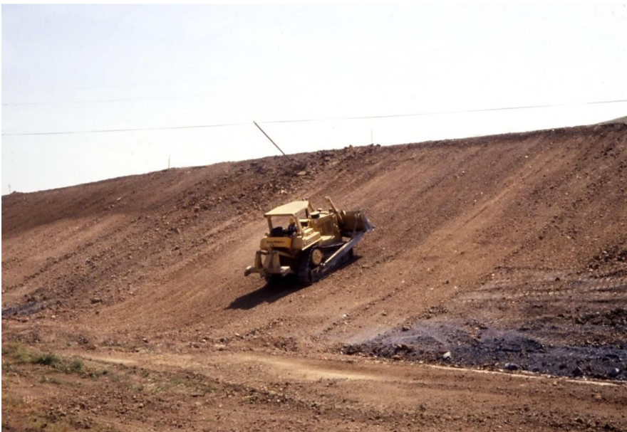
Figure 2-3: Illustration of the 1:3 slope fall
