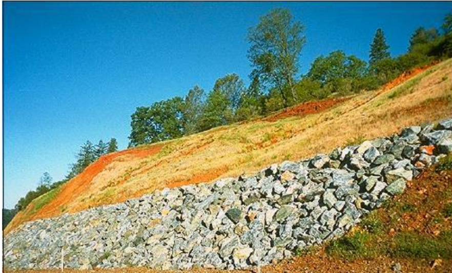
Figure 2-3: Rock buttress illustration
