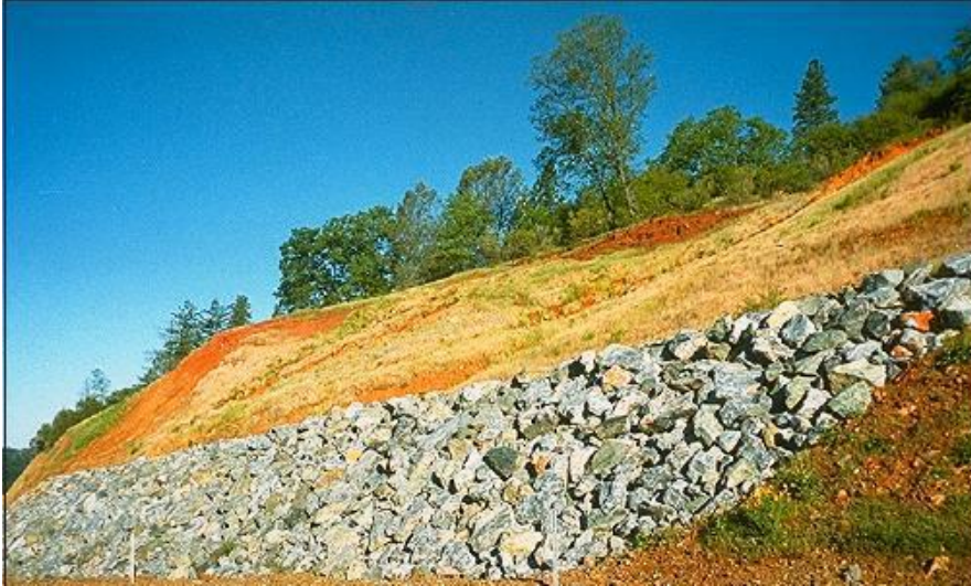
Figure 2-3: Rock buttress illustration
