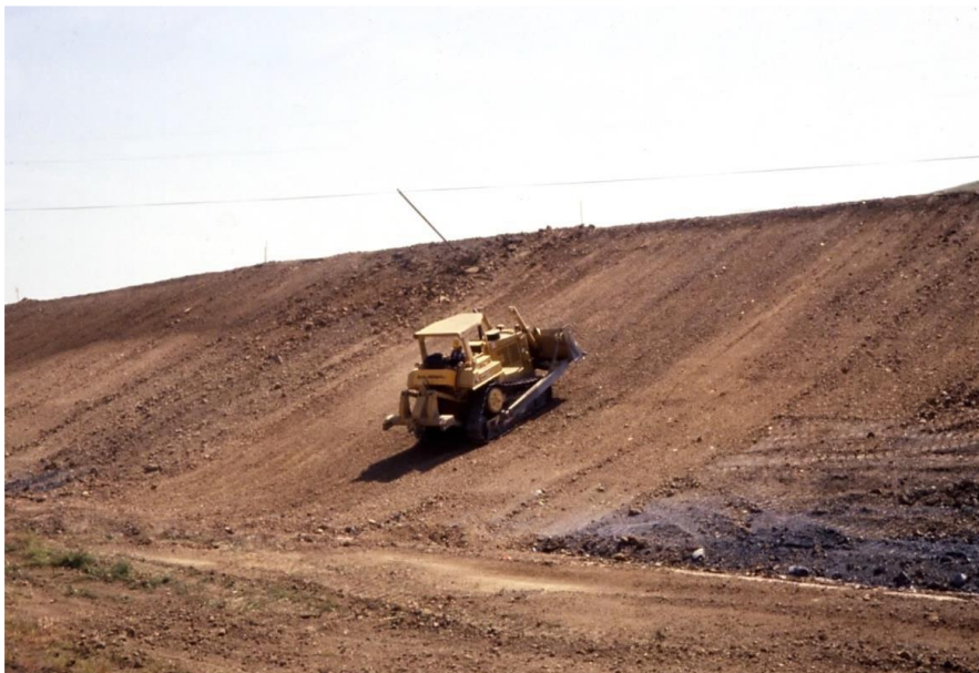
Figure 2-4: Illustration of the 1:3 slope fall
