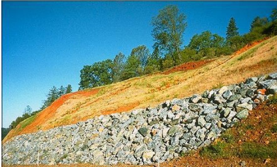
Figure 2-3: Rock buttress illustration
