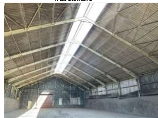
Photo 4-3 Cut-out of the roof
