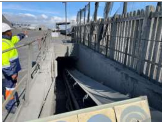
Photo 4-9 Conveyer line going underground
