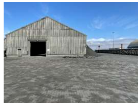
Photo 4-1 Outside view of the warehouse
