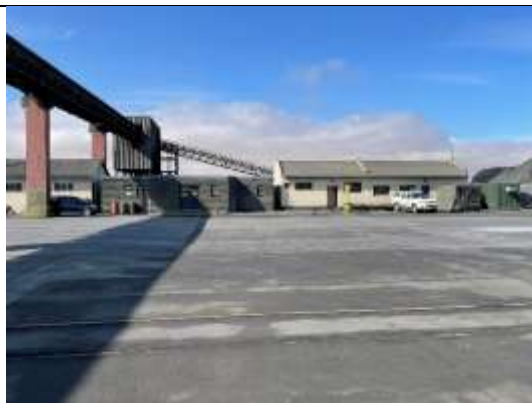
Photo 4-7 Conveyer line crossing the road towards the storage area
