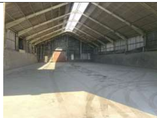
Photo 4-2 Inside of the warehouse
