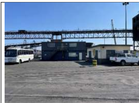
Photo 4-11 Office building and containers converted to office spaces
