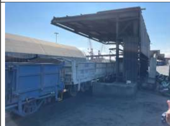
Photo 4-17 Rail way weigh bridge
