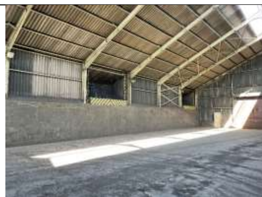
Photo 4-4 Loading bays located in the warehouse
