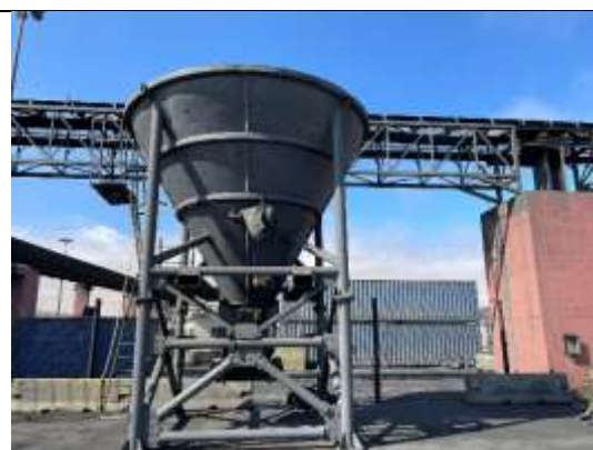
Photo 4-16 Hopper used to funnel the bulk cargo at the port
