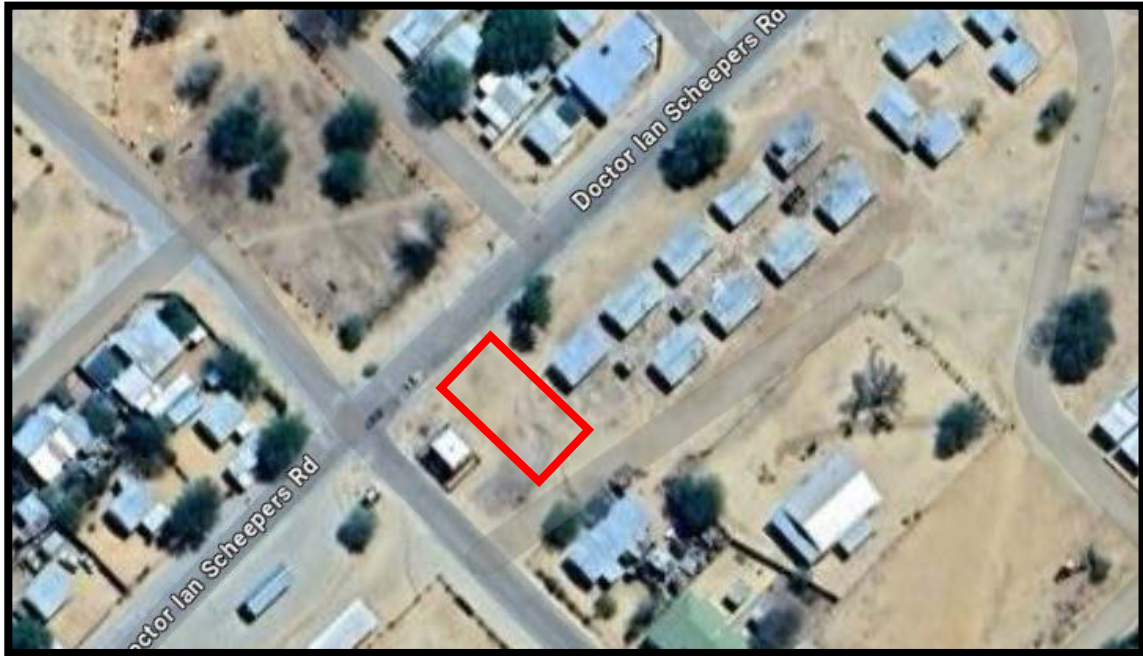
Figure 1: Aerial View of Erven 457 and 458 Ozondje
