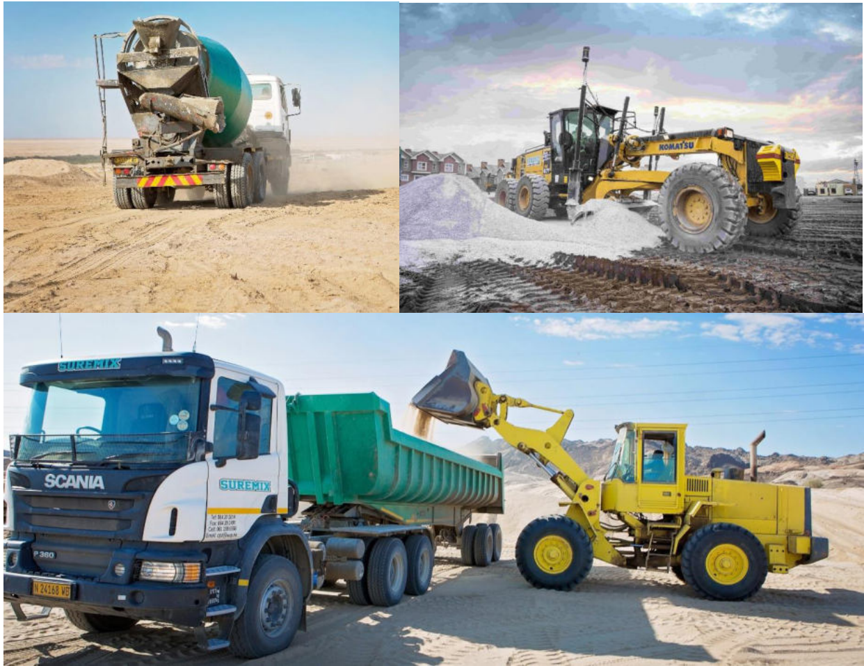
Figure 4: Typical Plant and Equipment of CPP Sites
