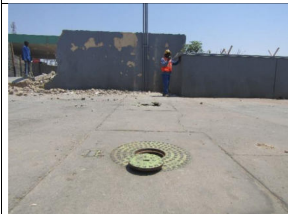
Image 3: concrete slab around the tanks filler area.
