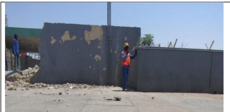
Image 1: Vent pipes have been installed on site (3m) to release vapors above the immediate atmosphere to enhance pollution attenuation.
