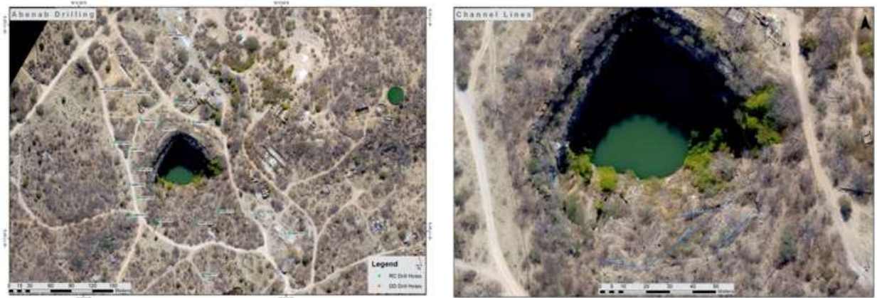
Figure 7. Drilling sites and Channel Line around the old Abenab open cast.
