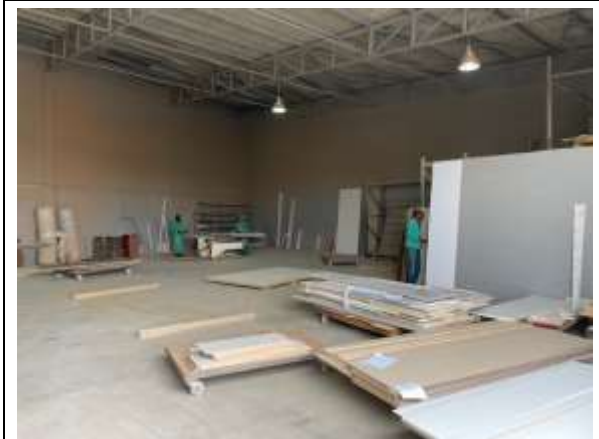
Photo 4-10 Interior of warehouse A
