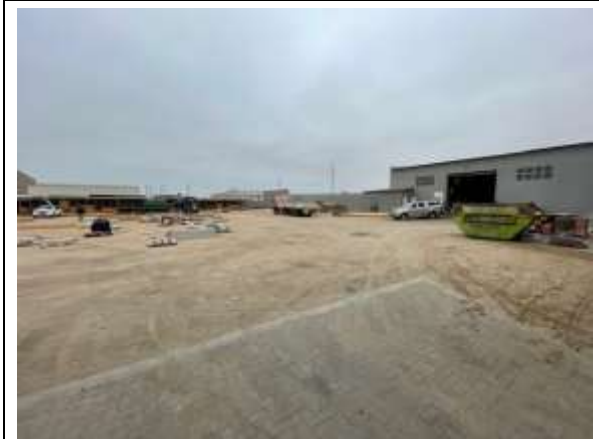
Photo 4-8 View towards the northern corner from the warehouses
