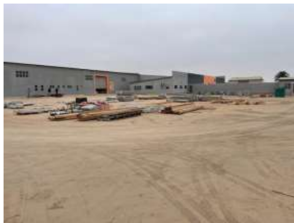
Photo 4-3 Outside view of warehouse D from the centre of the yard
