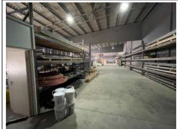
Photo 4-16 Interior of warehouse C and D from warehouse D's entrance
