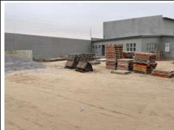
Photo 4-5 Back corner of the property with the ablution facilities
