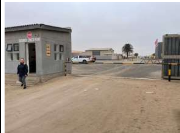
Photo 4-4 Main entrance with security office
