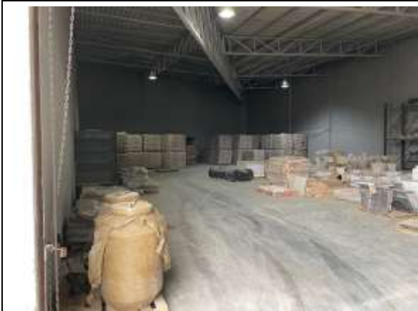
Photo 4-11 Interior of warehouse B
