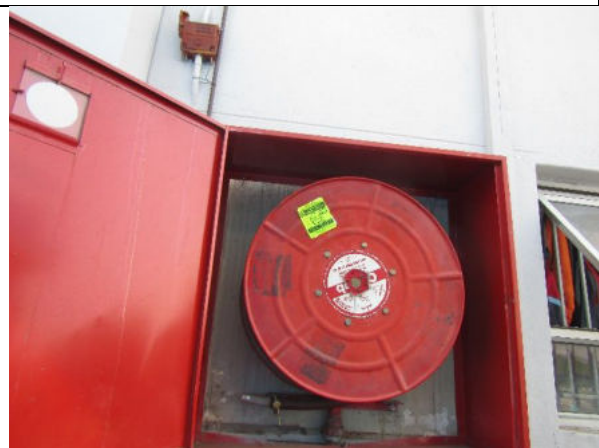
Image 4. Hose pipe on site
