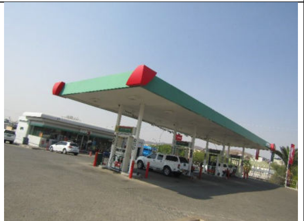
Image 4: Interlock surrounding the site
