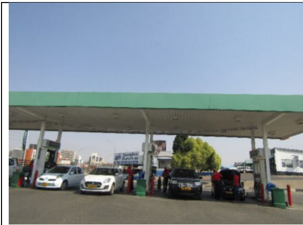
Image 1: A Canopy installed on site
