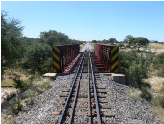
Photo 3.1.4 - Epako River Bridge
