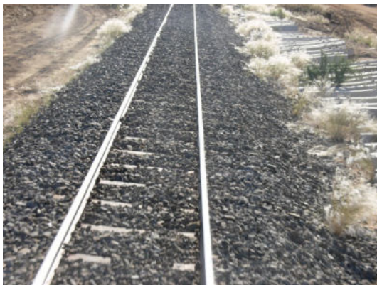
Photo 3.8.2 – Original steel sleepers
