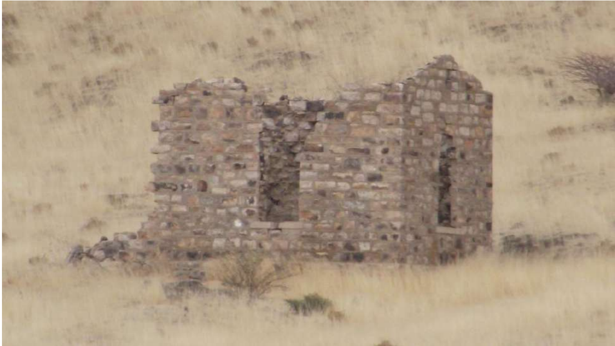
Figure 12; A ruined building structure (source: Authors 2022).
