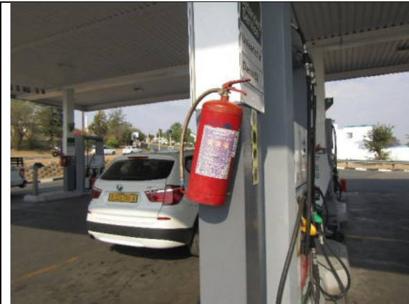
Image 1: one of the fire extinguishers on site.
