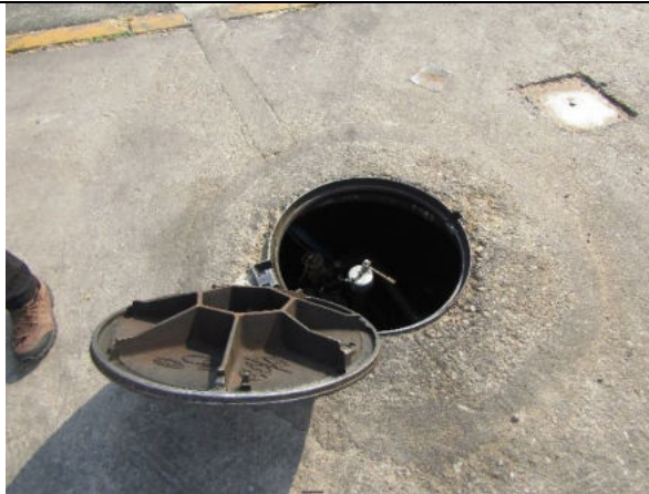
Image 1: Oil and water interceptor to collect wastewater and oils from the forecourt to the water and oil separator pits
