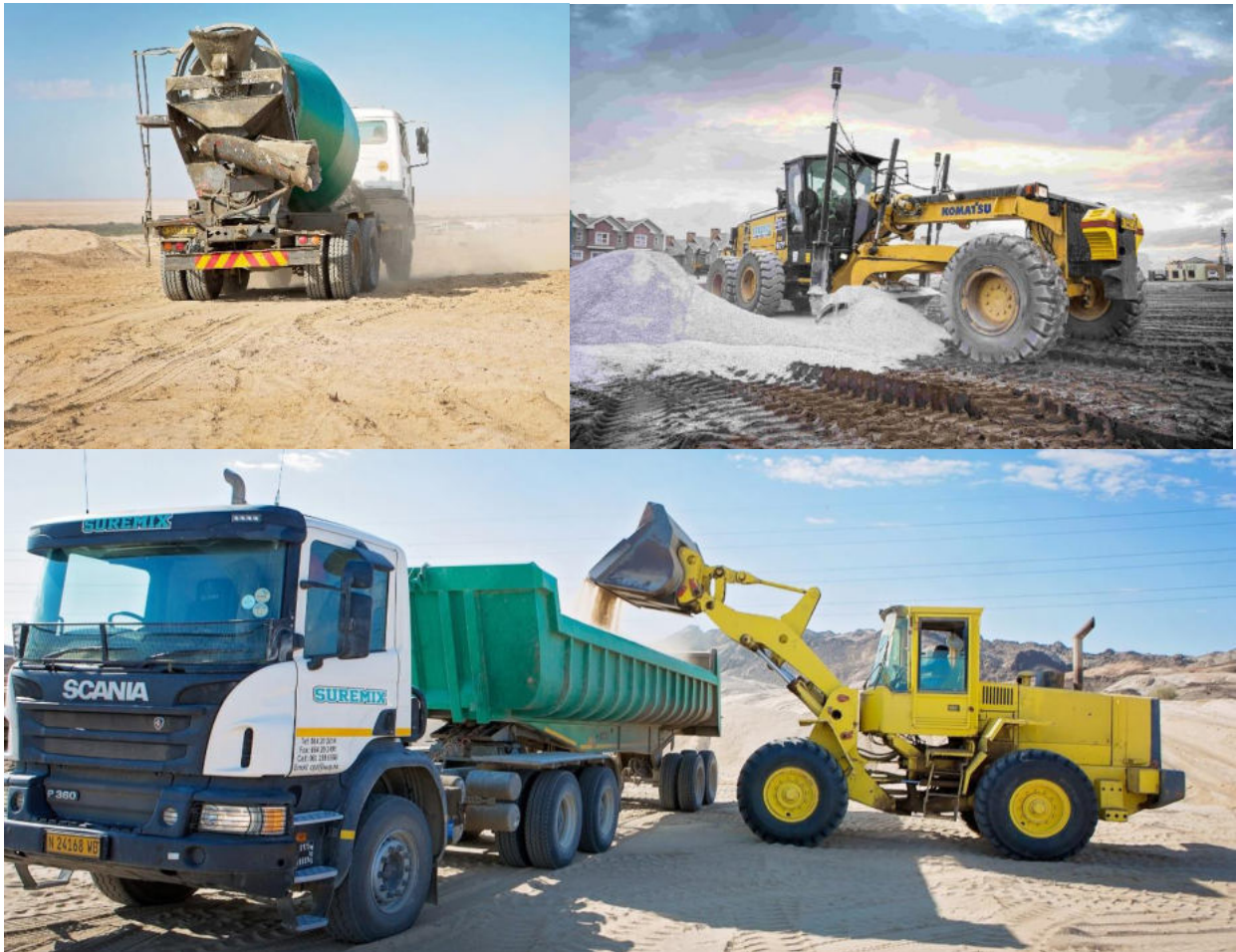
Figure 4: Typical Plant and Equipment of CPP Sites
