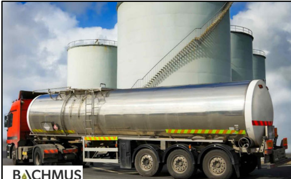
Figure 5: Fuel Supply tank
