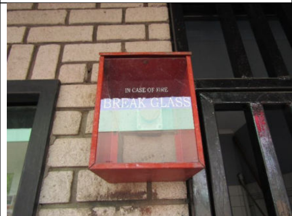
Image 4: emergency shutdown fire alarm
