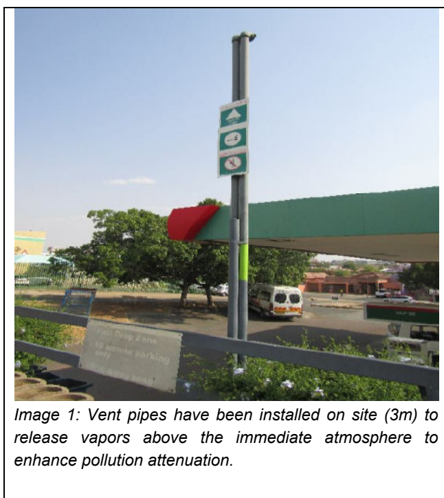
FIGURE 3: HYDROCARBON VAPOURS AND ODOURS POLLUTION CONTROL MEASURES CURRENTLY ON SITE
