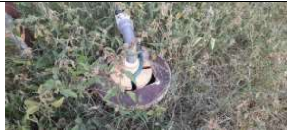
Photo 4-33 Borehole installation for domestic use ( WW39288)
