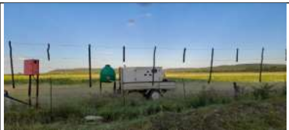
Photo 4-8 Mobile mixing unit
