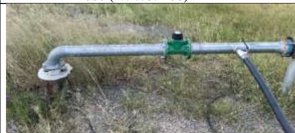
Photo 4-35 Borehole installation for irrigation use ( EB4 New Borehole)
