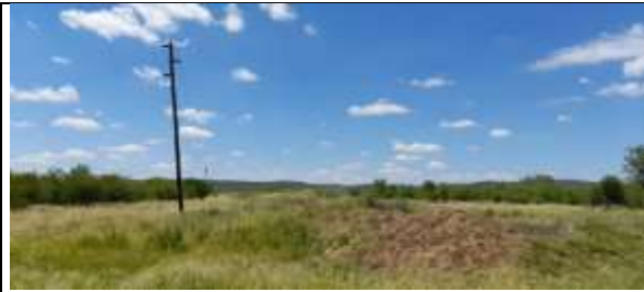
Photo 4-19 33 kV power line on site
