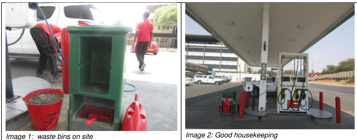
Figure 4: general waste pollution control measures currently on site
