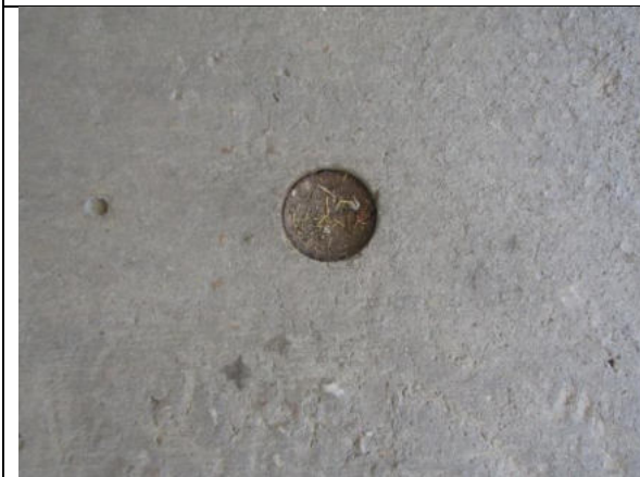
Image 3: Monitoring well on site.
