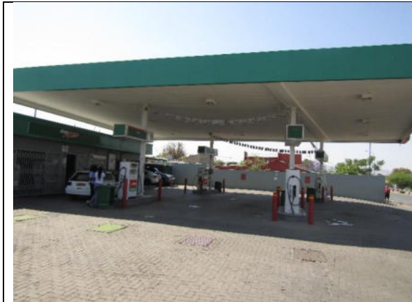
Image 1: A canopy installed on site.
