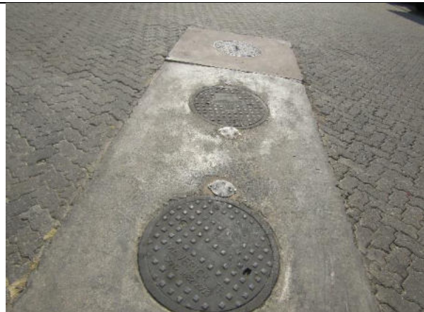
Image 2: Oil and water separator pits emptied regularly by certified contractors.
