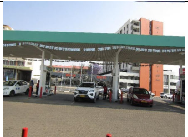
Image 4: Interlock surrounding the site
