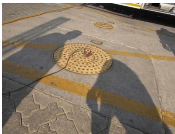
Image 2: A concrete slab around the tanks filler area and fuel dispensing points for surface spills containment.
