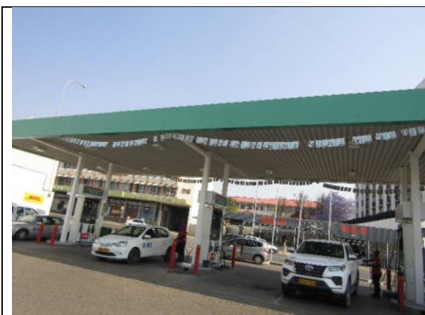
Image 1: A Canopy installed on site
