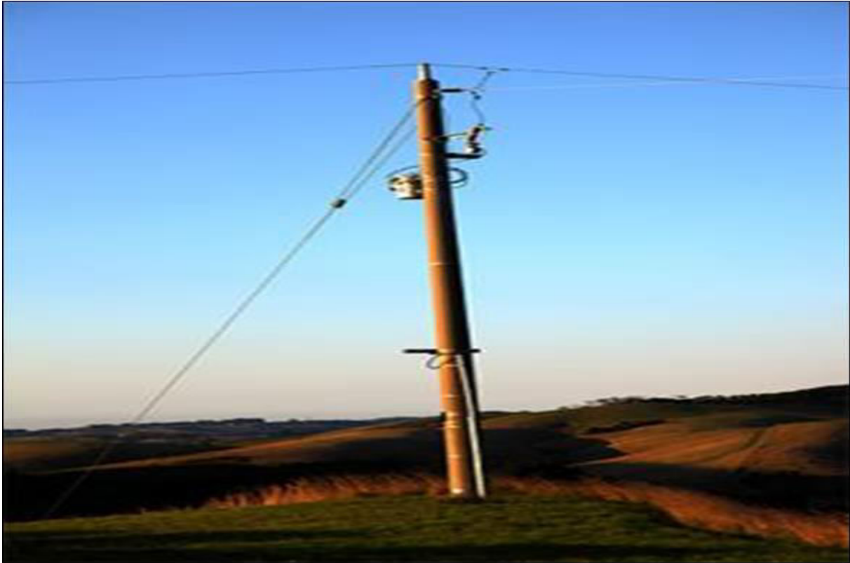
Figure 2: Typical single-phase design
