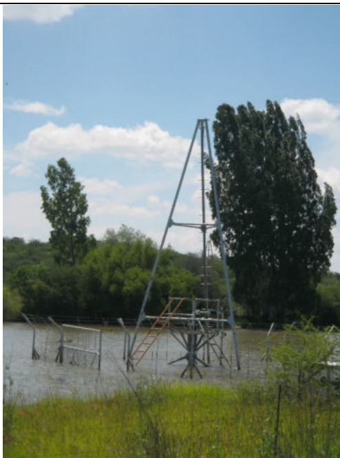
Photos 5.3 – View of a borehole located within the Kamanjab Dam
