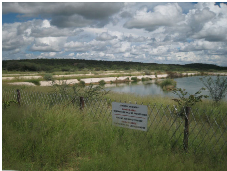
Photo 5.6 – View of Oxidation Ponds
