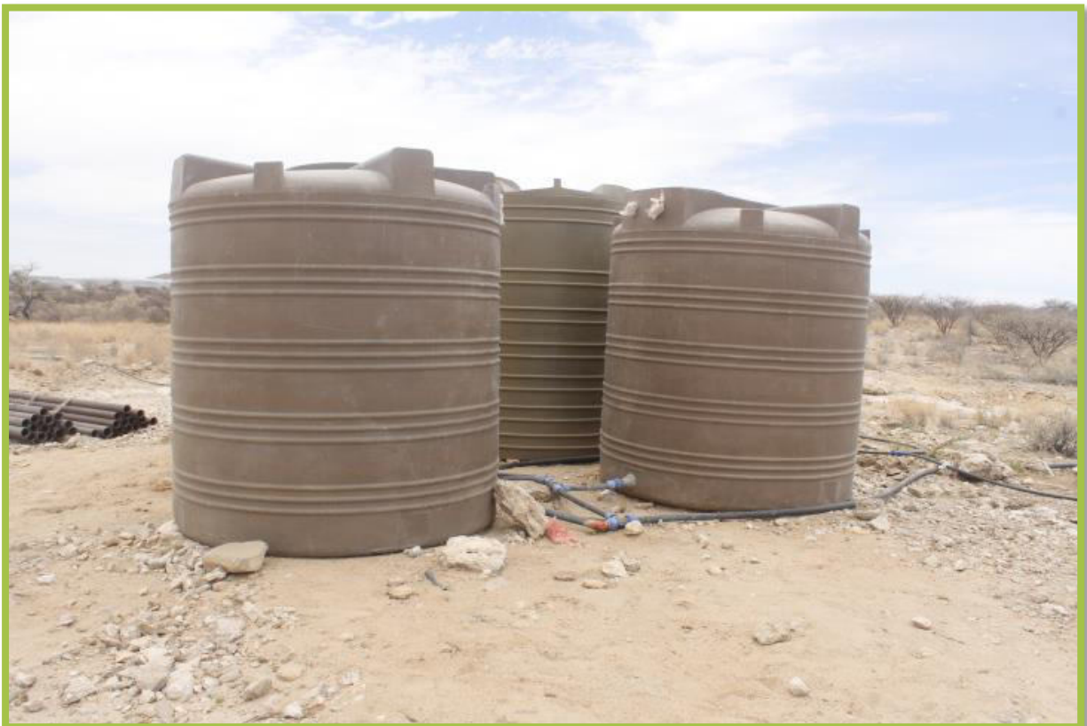
Figure 5: The 10 000 litres water tank that will be used for water storage during the operation of the mine.
