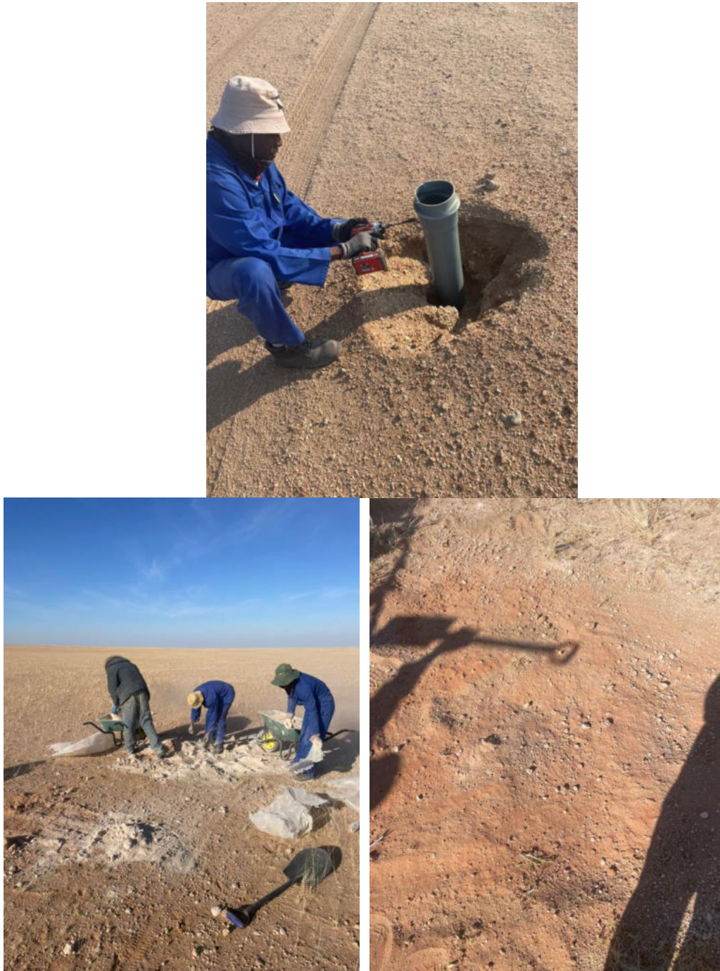
Figure 4 - Rehabilitation of holes drilled
