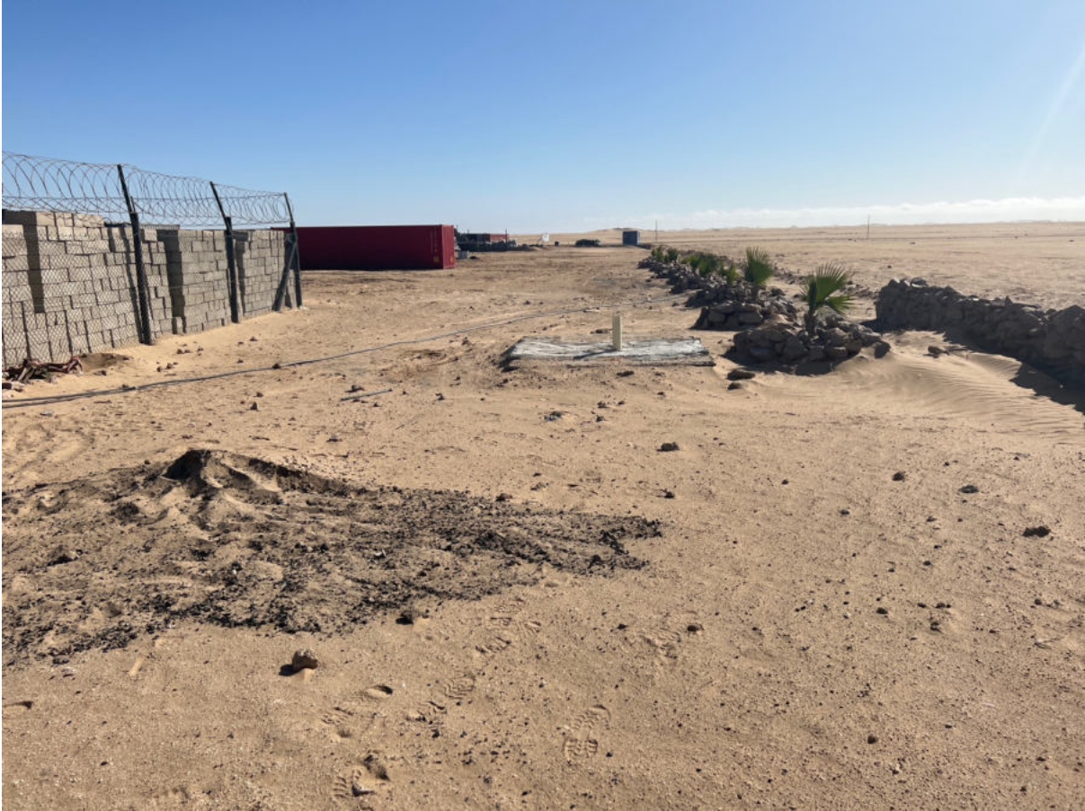
Figure 6: Septic tank wash away system used on site.
