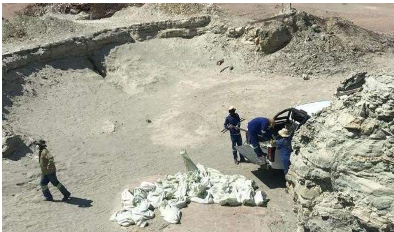
Photo 3 , Old Khan Mine surface dumpsite during reclamation recovery of ore on the site.
