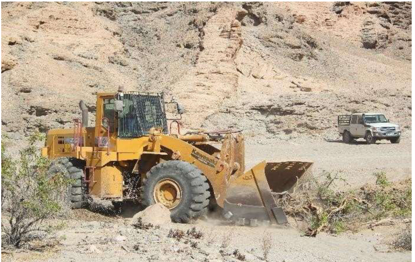
Fig 5 , Earth moving equipment clearing the way for access road.
