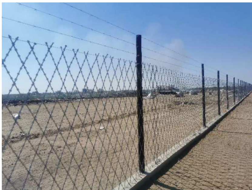
Figure 2-4: A view of the security fence around the site (eastern side)
