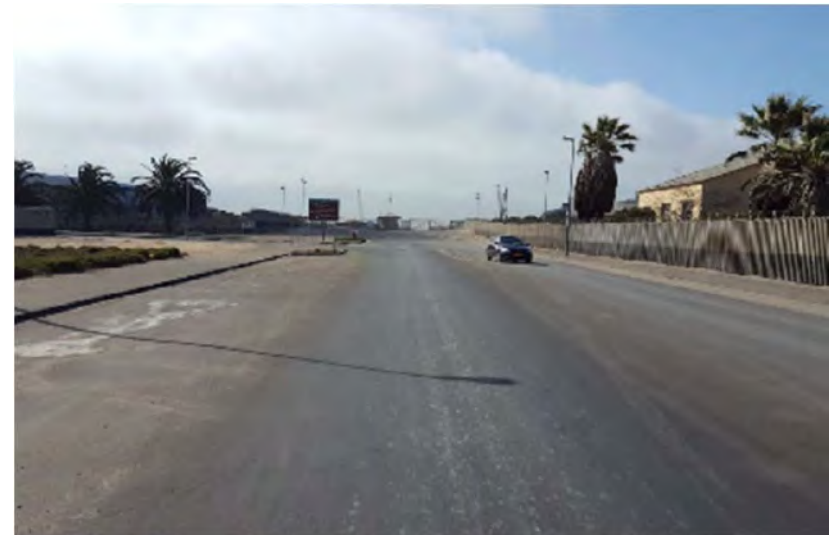
Photo 4: North-Westbound View along 5 th Road approaching Atlantic Street
