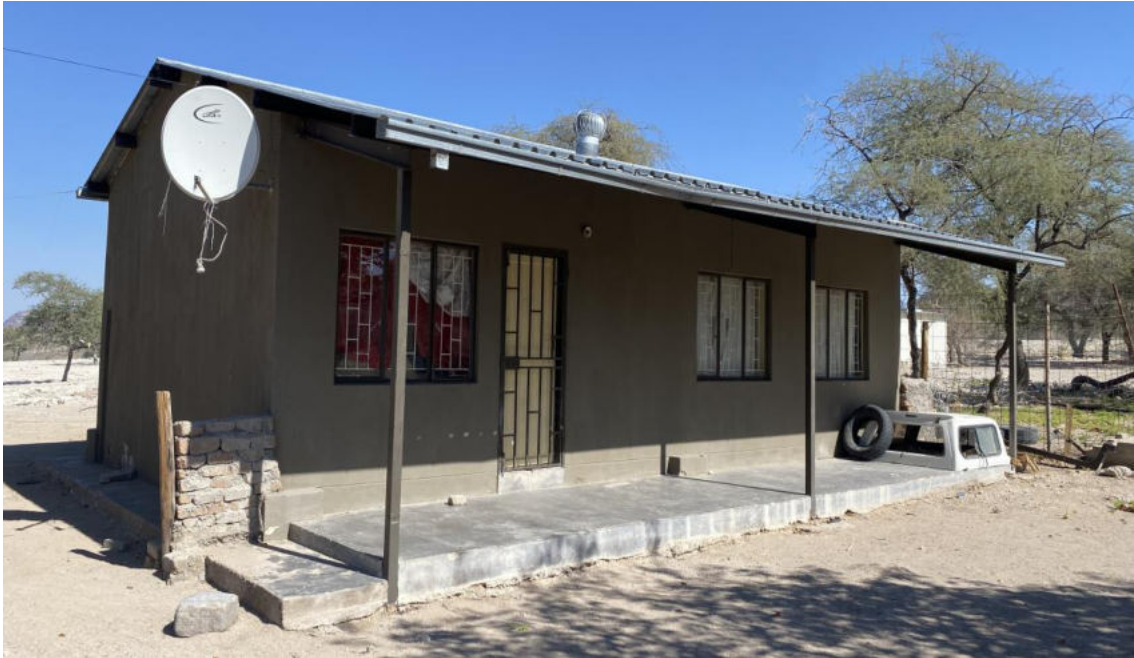
Figure 2-4: One of the three old brick houses at Sesfontein APU camp
