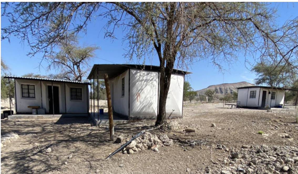
Figure 2-5: Three Barvaria units, which serve as accommodation for some of the APU members
