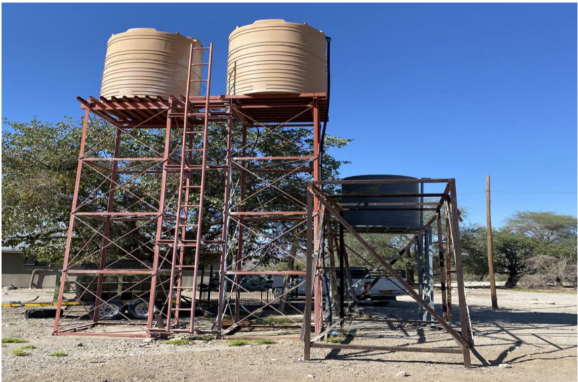
Figure 2-6: The two 2500 litres water reservoirs at the Sesfontein APU camp
