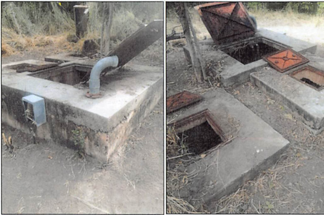
Image 6-1: Old Sewer System at the Project Site
