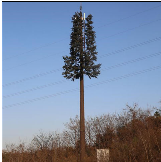
Figure 2: Typical example of a camouflaged telecommunication tower structure
