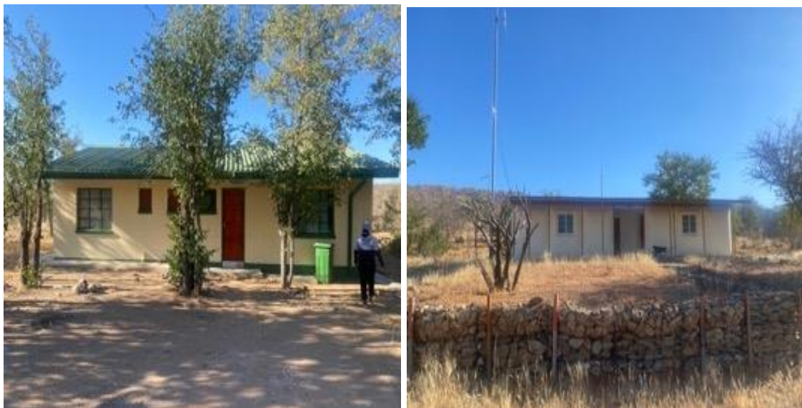
Figure 2.2: One of the renovated staff house (left), and office block (Otjovasandu A).
