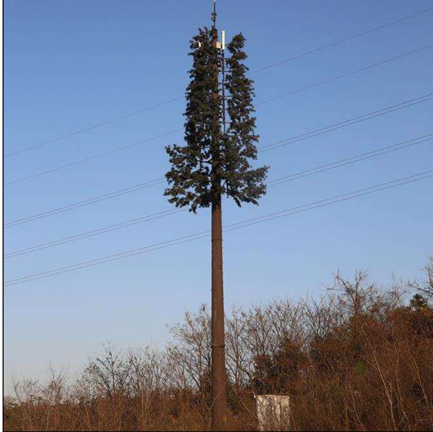
Figure 2: Example of a camouflaged tree telecommunication tower
