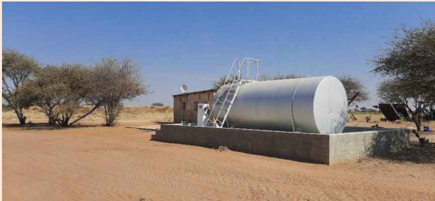
Figure 6: Pictures showing: a) the new fuel installation; and b) cracked bund wall (Source: L. Maartens, 18 July 2024).
