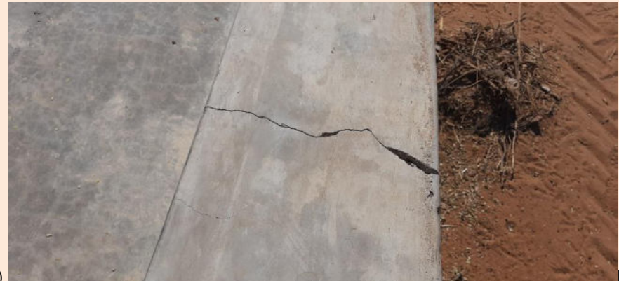
Figure 6: Pictures showing: a) the new fuel installation; and b) cracked bund wall (Source: L. Maartens, 18 July 2024).
