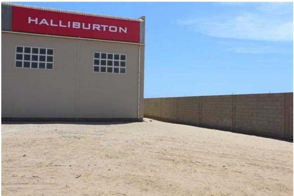
Photo 5-5 Proposed location of the radioactive bunker
