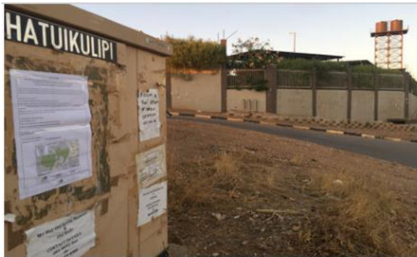
Tauno Hatuikulipi Substation
