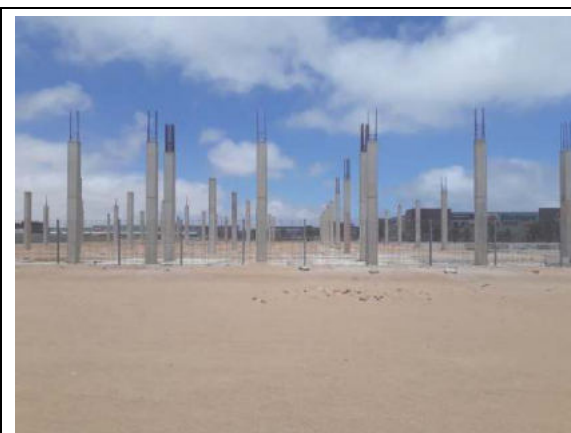
Photo 7-2. Southern neighbour (Van der Walt Transport future copper storage warehouse)
