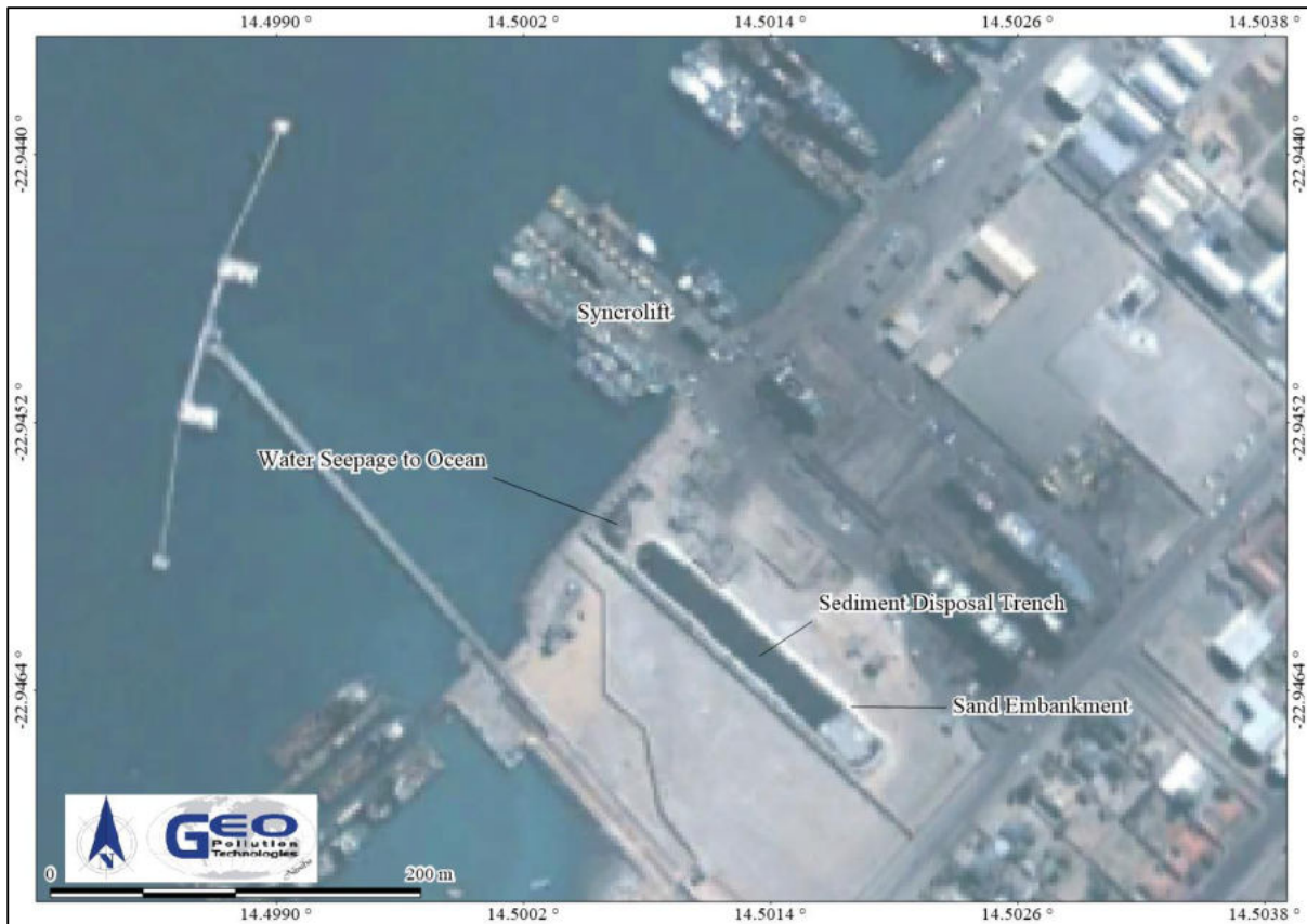
Figure 6-4 Onshore disposal site (Google Earth 06/2007)
