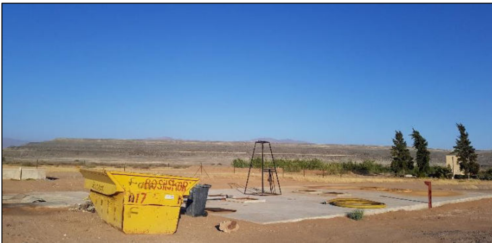
Figure 4: Sewage collection point (to sort out any solid wastes)
