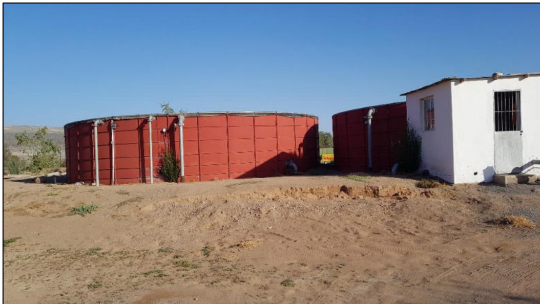
Figure 7: Storage Tank for treated water
