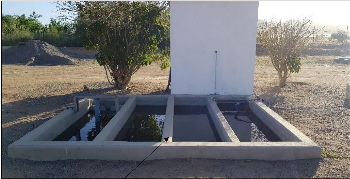
Figure 8: Chlorine dosing dams
