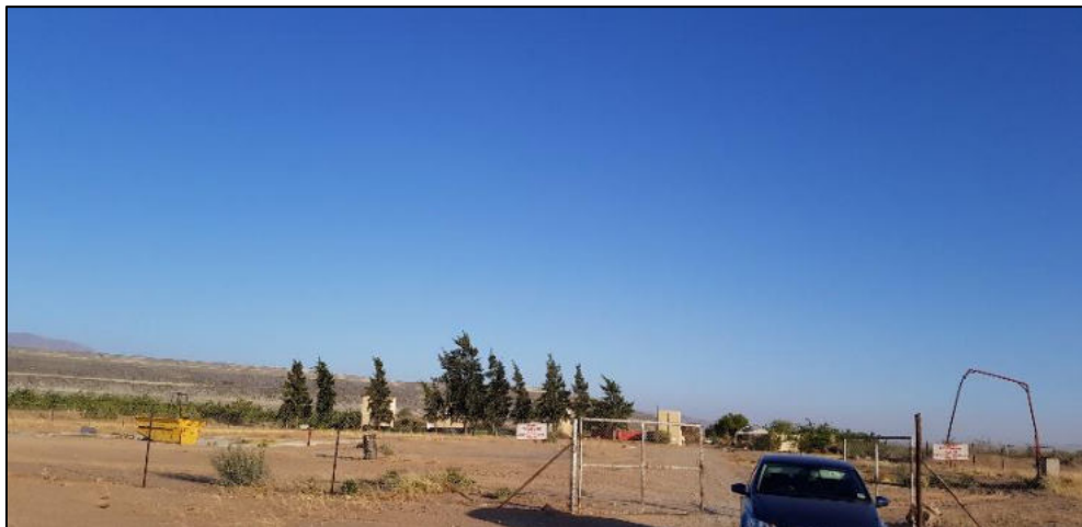
Figure 5: Entrance gate to the Sewage Treatment Plant
