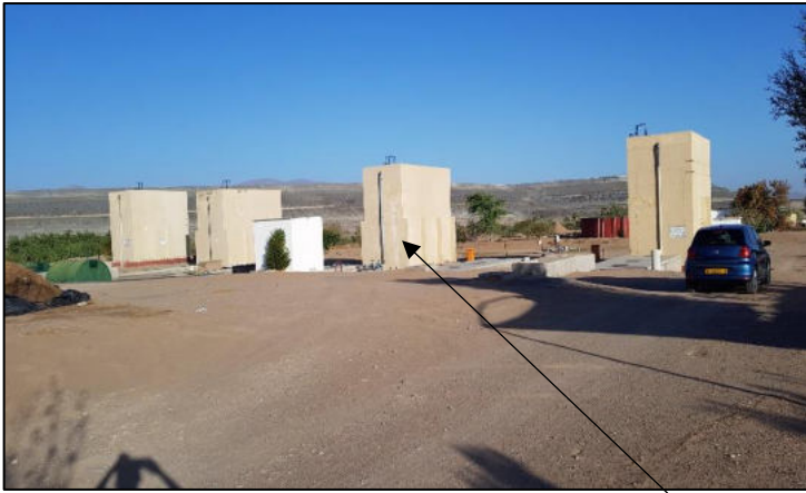
Figure 3: Trickling Filter Towers
