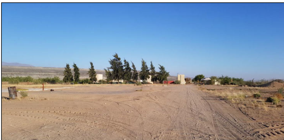
Figure 2: View of the Sewage Treatment Plant site
