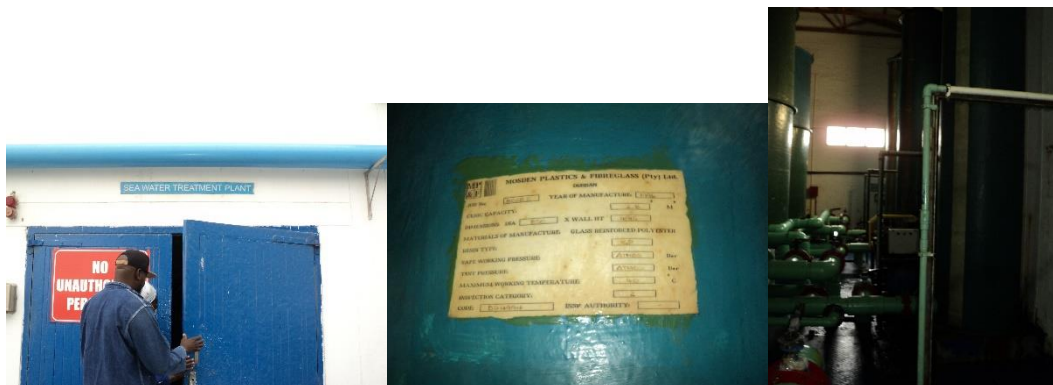
Plate 5: Pumping of filtered seawater into four (4) flocculation columns at 120 m 3 .
