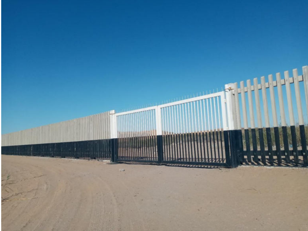
Figure 1: Completed fence at the entrance of the landfill site, phase 1 and 2
