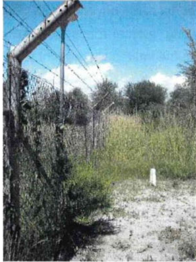
Figure 18: Electrified 2.4 m high predator proof fence at Shisinze Station (source: LCE)
